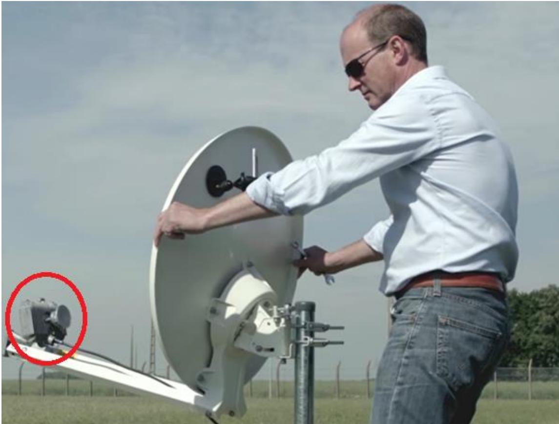
When aligning the dish, start by checking the elevation results and adjust the dish bracket accordingly.
